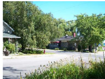
Address: Approximately 131 Nagonaba Use: Commercial/Retail “The Depot” Style: Stone Train Depot Contributing: Historic-Yes Architectural-Yes
