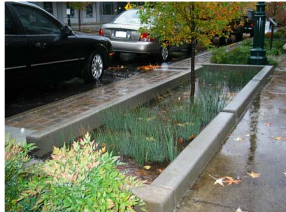
Storm-water planters integrated into redeveloped streetscapes in Portland, Oregon—are possible for parts of Nagonaba Street
