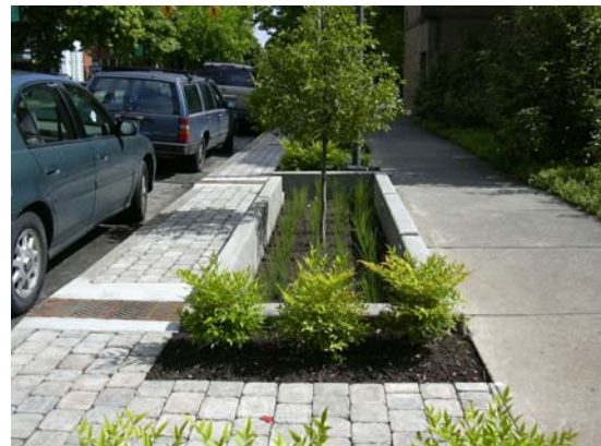
Storm-water planters integrated into redeveloped streetscapes in Portland, Oregon—are possible for parts of Nagonaba Street
